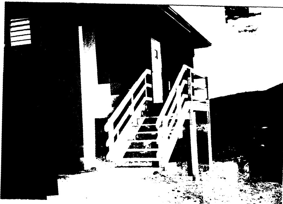
Figure 1. An emergency exit at the St. Thomas Community Rehabilitation Center that leads to stairs rather than to a wheelchair ramp. (Office of Inspector General photo)
